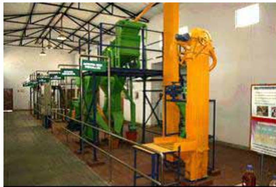
Pilot plant for Bio Diesel at AAU Anand
