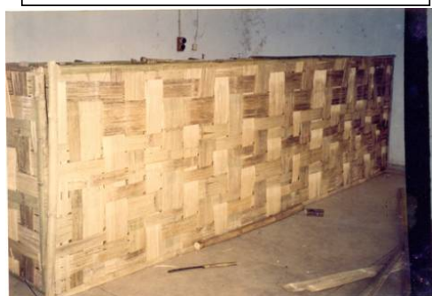
Double Wall Bamboo Structure
