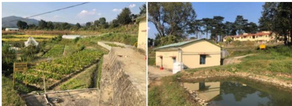
Rain water harvesting cum gravity based micro irrigation system
