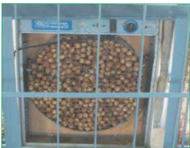
Fig. 17. Desiccant wheel fitted on the evaporative cooler
