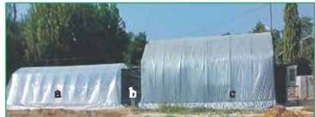
Fig. 71. (a) Compost pasteurization unit (b) Passage (c) Mushroom production unit
