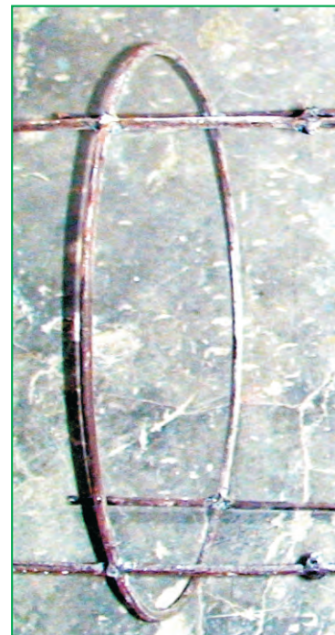
Fig. 49 View of ring and bars placed inside the concave
