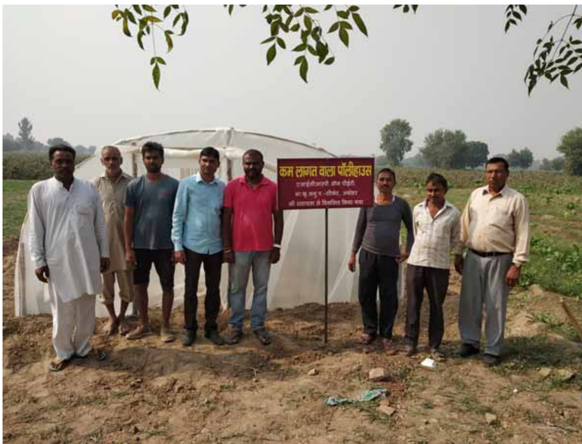
AICRP on PET, ICAR-CIPHET Abohar constructed four low-cost polyhouse structures (floor area 60 m 2 ) at farmers' fields in the village of Amarpura and Kala Tibba
