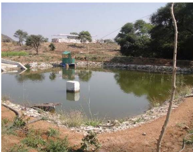
Fig. 57. Plastic lining of water harvesting tanks
