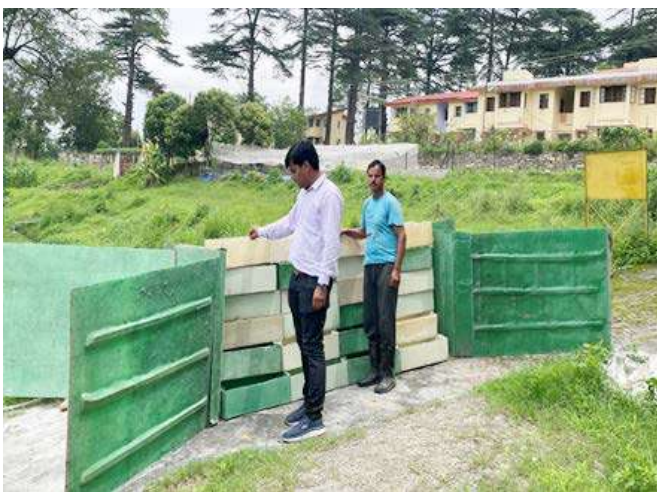
Fig. 48. Plastic Check Dam for Water Management in Hilly and Semi-arid Region
