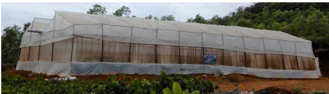
Fig. 2. Bamboo polyhouse (designed wind speed: 100 km/hr, Area: 528 sq.m, Gutter height: 4.57m) erected at farmers field
