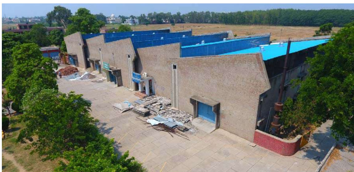
Renovated Workshop Building at ICAR-CIPHET, Ludhiana
