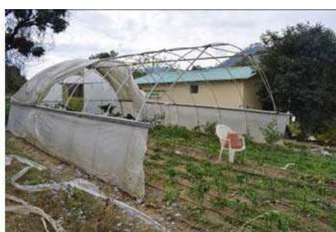
Dismantling & shifting the portable polyhouse
