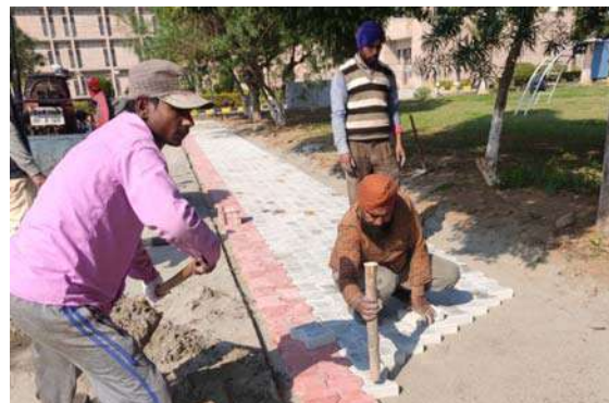
Interlocking Tiles work at Ludhiana campus
