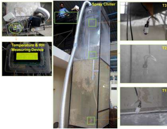
Fig. 58. Temperature and relative humidity measuring device used for real time-monitoring of spray chilling process
