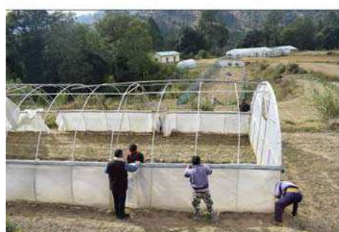
Fixing the window and middle parts in new field
